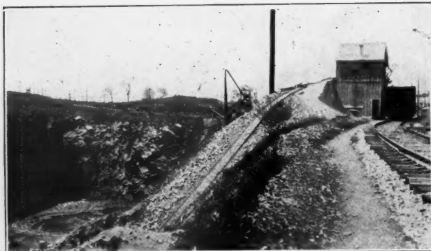
Top of Incline and Hoister House
